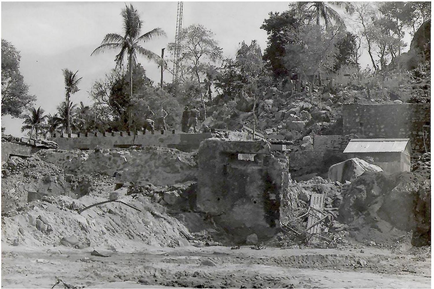
Ba Xoai after the January 1970 attack. This is the heavy inner wall by American SF area that has been destroyed. Outer walls already breached. A four-deuce and 105 Howitzer were destroyed
